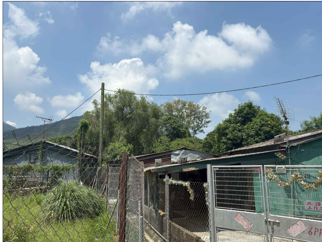
LR7 Workshops and Storage Yards
